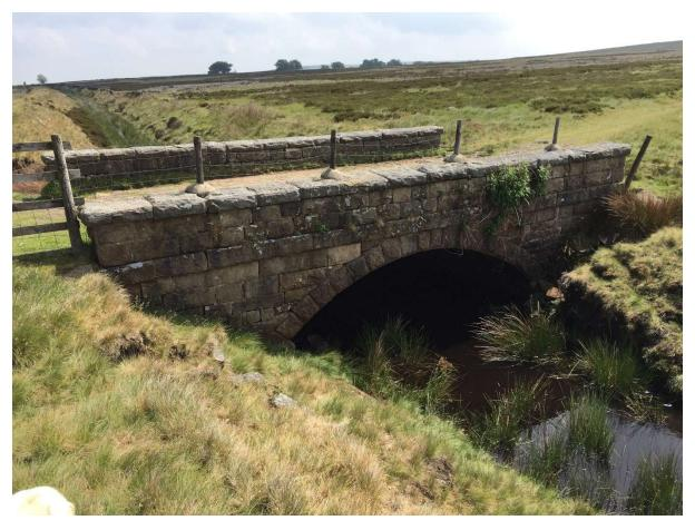
The conduit begins north east of Stanage Edge and captures water which would otherwise fall into the Rivelin reservoir, instead taking it to the higher Upper Redmires Reservoir and feeding into smaller supply reservoirs in west Sheffield.
