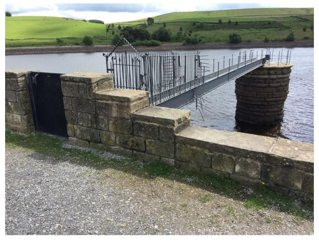
This is the outfall for a pumped water supply from the Rivelin Water Treatment Works, raising clean water 120 metres to Redmires Lower Reservoir, after removal of peat and impurities.
