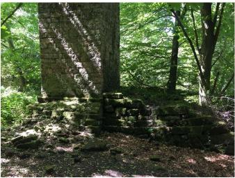
Stone built square chimney to take the smoke from the boilers used to heat Paxtons Great Greenhouse. Eight boilers heated water to keep the greenhouse hot. Cartloads of coal came across the moors and down zigzags within Stand Wood to deliver coal daily to keep the boilers going. 300 tons were needed in winter.
