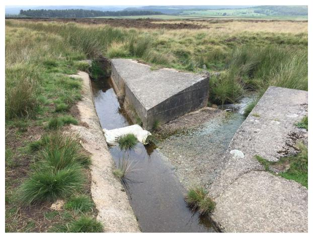
Umberley Well conduit supplying Swiss Lake, has a modern overspill weir allowing excess water to overspill and drain naturally across Gibbet Moor to join the Emperor Stream, and into the Emperor Lake.
