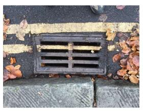
Nether Edge has a handful of remaining historic manhole and drain covers. This drain cover is from 1849 when drainage improvements were installed as part of anti-cholera measures. The inscription is too worn to be legible, having been run over by steel rimmed wheels for many years. Many have been stolen for scrap metal value, and their replacements are cleared labelled 'Non Metallic'
