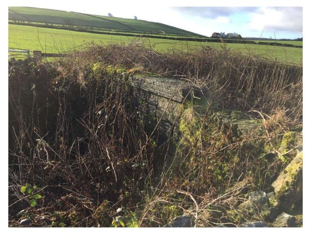
Water from the Redmires Reservoirs was led into Sheffield by a small conduit which sliced through enclosed fields. Sheffield Water Works had to erect crossing points for farmers. This is one of many small bridges. The bridge width was adequate for horses and oxen with ploughs, but not wide enough for the tractors and ploughs which were soon to follow.
