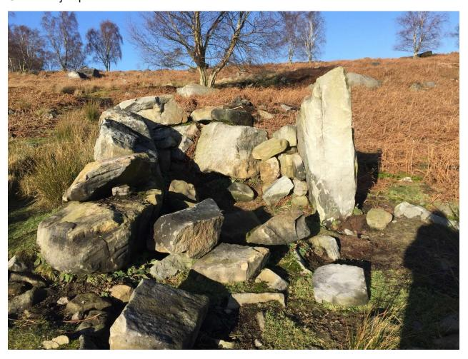
One of a line of 8 shooting butts below the track leading to Wharncliffe Lodge. Not so much 'built' but 'assembled' by a large earthshifting machine using massive boulders gathered from the surrounding Moor. More like a megalithic monument than a shooting butt.
