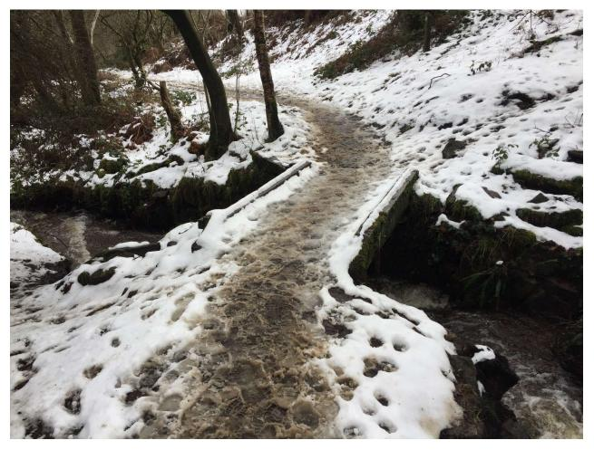
These small bridges are regularly destroyed by flooding. The Limb Valley drains quickly and flash floods overtop the steam banks, washing trees and boulders downstream. These block at the bridges which eventually collapse.
