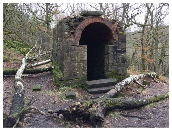
This solid stone walled small building with a barrel vaulted brick roof is a long way from anywhere. It might have been an explosives store. There are no windows but plenty of ventilation. Explosives were used in the building of the Totley Tunnel, and in the Bolehill quarries.
