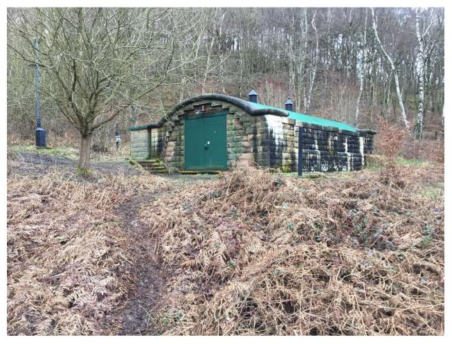
A well known building at the edge of Upper Padley at the entrance to the dramatic scenery of Padley Gorge. People recognise it as something to do with the water pipeline but most think it's a pump-house. It is actually a remotely managed valve house, enabling the flow in the pipes to be adjusted according to demand. It has the same green paint as other Derwent Valley Water Board metalwork, and a very attractive barrel-shaped roof.
