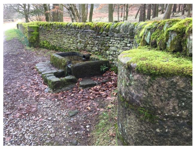
A well built arrangement of small millstones as buttresses built into the dry stone boundary wall to create a small embayment.
