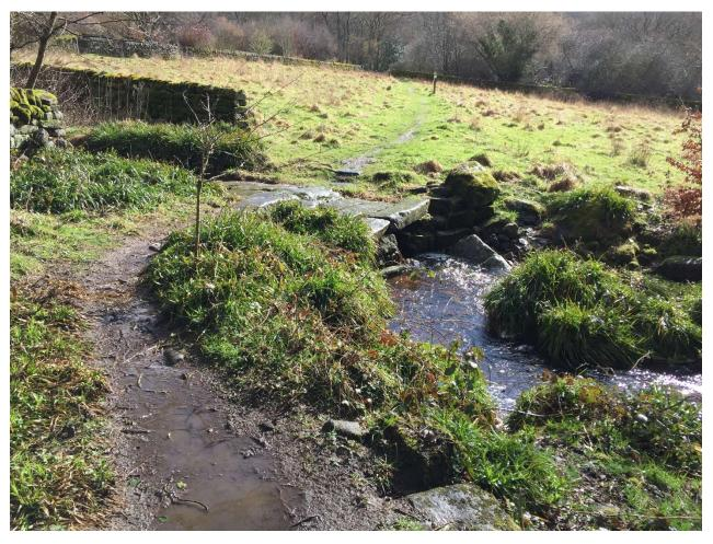
Pairs of heavy duty gritstone planks span the stream. A central wall supports them. They extend upstream well beyond the width needed to allow a cart to cross, some five metres.
