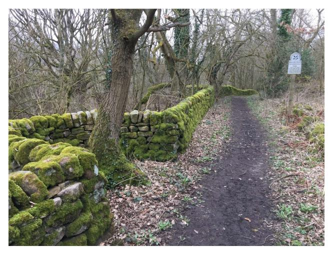
Just inside the top gate to Froggatt Wood. One of two semi-circular wall embayments built around small trees. There are no other embayments in this wall, just these two about 50 metres apart on the flat top length of track.
