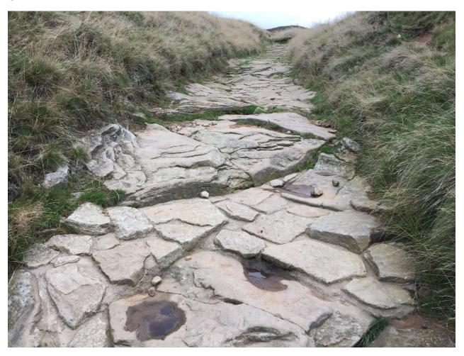
Years of packhorse and cart use has cut Chapel Gate down to the gritstone bedrock. 4WD vehicles finished the job and exposed the bedrock. Some infilling of the worst poyholes has improved the surface for mountain bikers.
