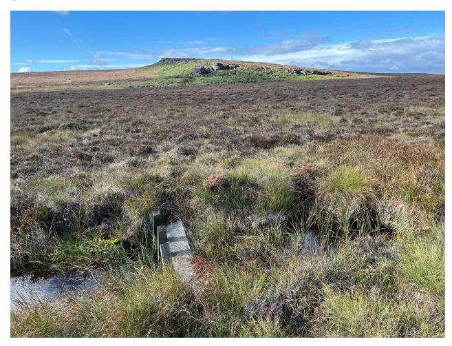
In recent years the Eastern Moors Partnership have introduced a new practice of slowing down water drainage from the moors. They have created a series of mini-dams of varied construction which attenuates flow. This timber staked dam has a nominal pedestrian bridge. There have been unfortunate spills from previous timber bridges which eventually collapse and dump the user into the dirty water.
