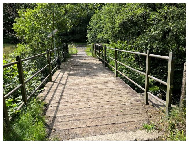
Haggwater Bridge is the last crossing point over the River Ashop before the Ladybower Reservoir. It is built high above the river because very high volumes of water are carried after rain, and lesser bridges have been washed away.
