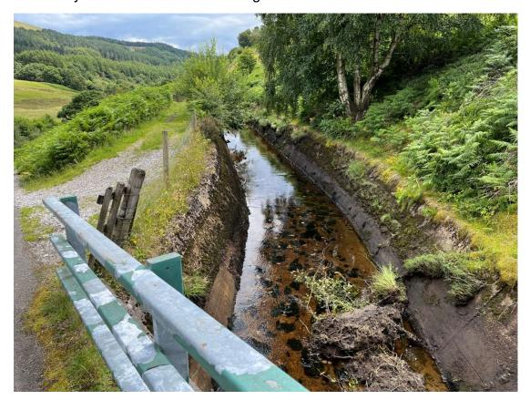
The River Ashop is 'captured' just above the junction with the River Alport; water follows in a concrete channel which drops down into a gravity fed siphon with a pipe bridge over the bed of the River Ashop. The siphon pressure pushes the water up the other side, then through a 1.8 metre diameter 975 metre long tunnel which discharges the captured water into the Derwent Reservoir, above Fairholmes.
