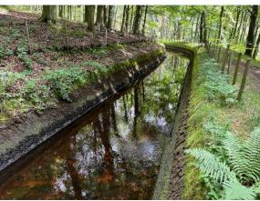
The Ashop Conduit is a concrete lined gravity fed channel which flows under Hagg Side.
