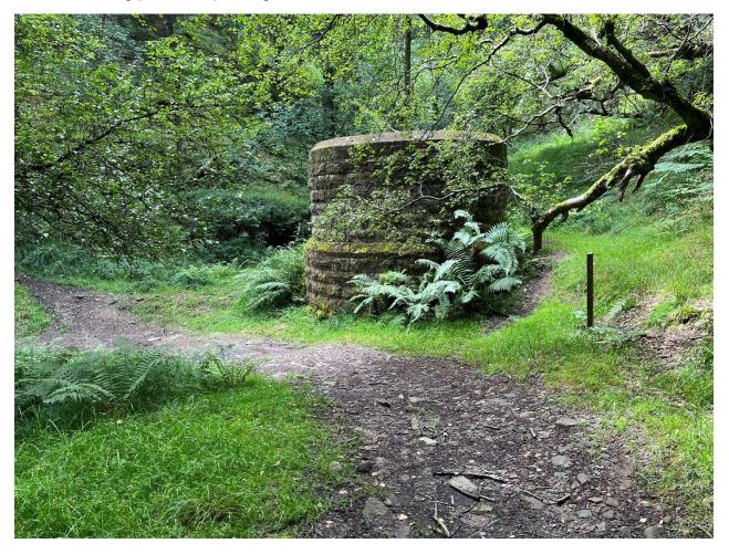
This stone chamber has a ladder and locked manhole cover on top. Possibly part of the Ashop Siphon, a spillover for excess water to be returned to the River Ashop.
