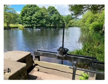
A crossing point has been established here since 1782, now comprising a number of lightweight timber bridges on stone pillars, and a short section of 'stepping stone' planks supported by brick built pillars. The section of 'stepping stone' crossing is very short and it is said to be the easiest stepping stone crossing in Derbyshire.
