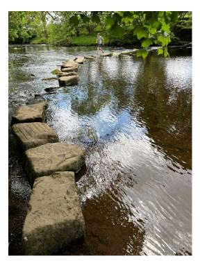
The stepping stones comprise about 30 massive stone blocks placed on the river bed. It times of high flow the stepping stones disappear beneath the river. At this point the River Derwent is 25 metres wide, and wading across would be dangerous.
