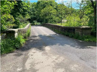
Notably this stone bridge has at least five metres clearance above the river in normal flow. The masons have clearly taken account of periodic flash flooding of the River Derwent.
