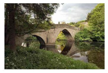
Froggatt Bridge is a narrow packhorse bridge with a pair of cutouts to allow laden horses to pass. It is unusual in having a large arch on the east Froggatt Village side, and a smaller arch on the west side. This may have been needed when the river was widened
