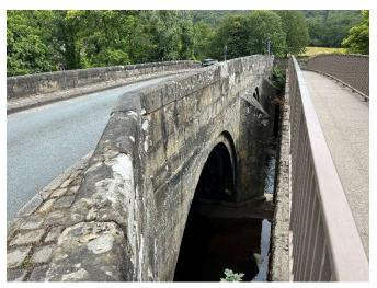
Grindleford Bridge is a three arch stone bridge with a more recent steel footbridge added on the downstream side. The bridge isnt wide enough for a footpath, so a similar arrangement to Mytham Bridge has been erected.
